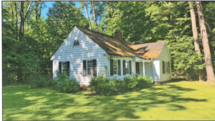
2. Looking south-southeast at the eastern house in the Building Area in the northeastern corner of the Protected Property.
