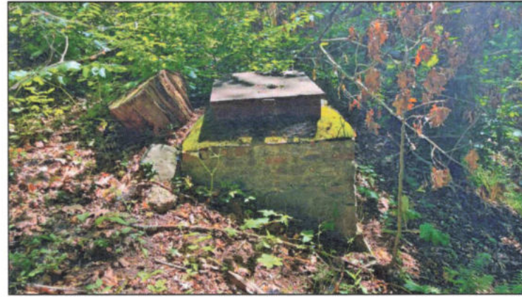
7. Looking east at a manhole for a water cistern located south of the eastern house.
