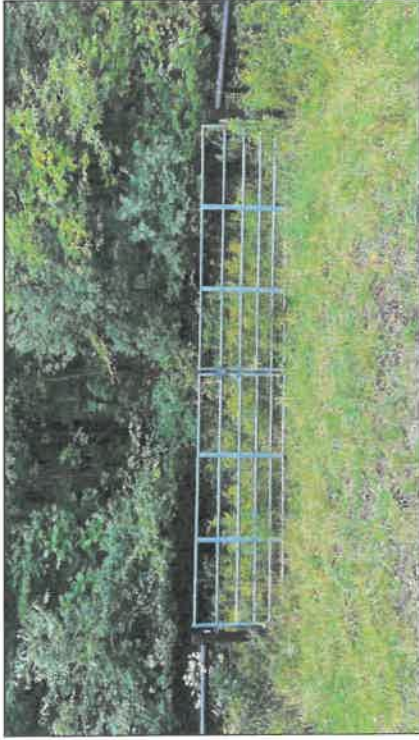
11. Looking west-south west at a gate in the fence that extends along the western property Boundary. Lake Metroparks owns the property to the west.
